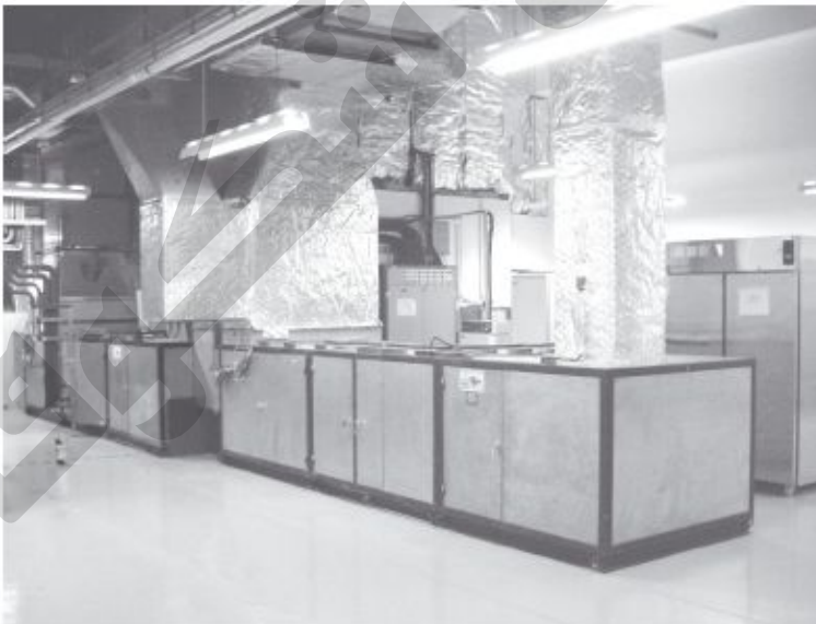
Figure 5.2 Cleanroom air conditioning plant
