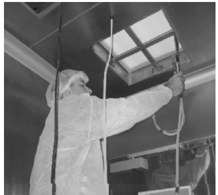
Figure 12: Measuring an air filter for leaks using a fish-tail probe.
