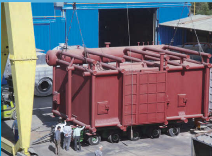
Mono Drum-Boiler: 50 Ton/hr SGG copyright November 2022
