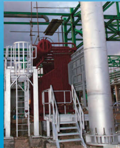
Mono Drum-Boiler: 2.5 Ton/hr
