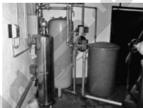
Figure 2.3 A water softener, showing the brine tank and microfiltration system.
