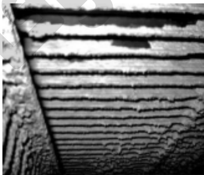
Figure 10.3 Scale in a tunnel pasteurizer.
